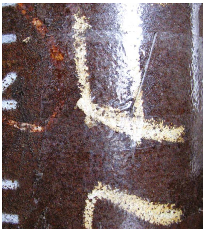
API 5L Piping
